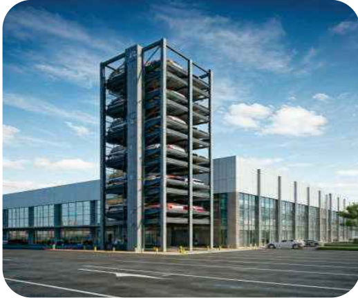
Multilevel Car Parking Systems
